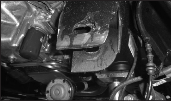
FIGURE 21C - DRIVER SIDE REAR
