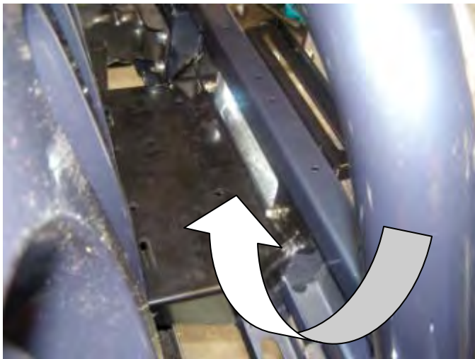
WINCH MOUNTING PLATFORM
