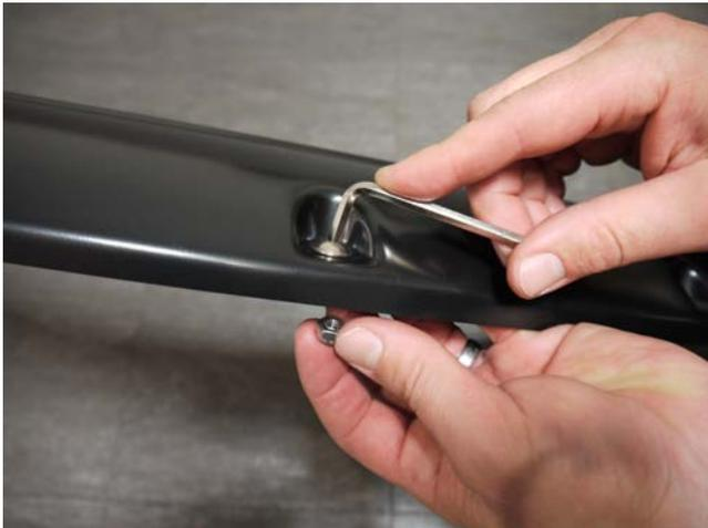
**STEP 7:** Attach the 11 bolts, washers and nuts to each Fender Flare using a 3/16" Allen key and a 10.0mm wrench/socket. (wrench/socket and Allen key not supplied). Ensure inside of Fender Flares where the rubber seal is attached is clean, using the alcohol wipes provided. Wipe away any residue with a dry clean cloth.
