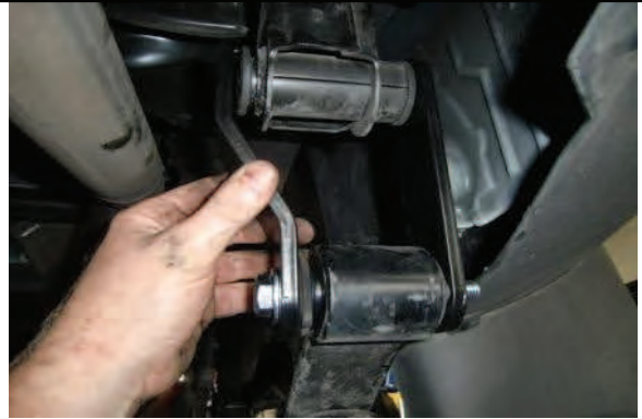
Attach new inner brackets and hardware
