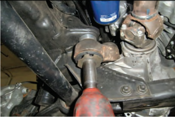
Install (4) differential drop spacers with new hardware
