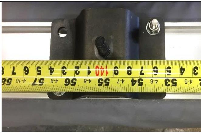
Install awning brackets on to awning and set at the required pitch taken from the previous step.
