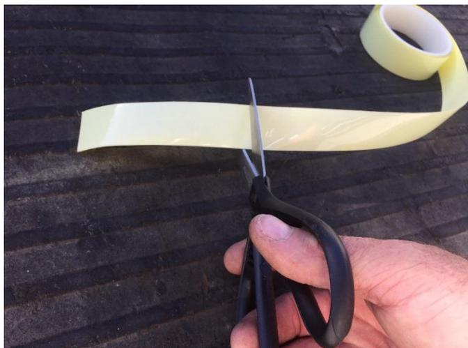
Cut 8 lengths of adhesive strip at 150mm each.
