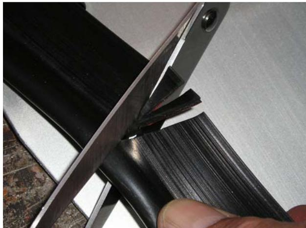
55. To fit rubber sealing strip to underside of aluminium step plate, lay strip on the underside of step plate and place so over hang is even on both ends. Using scissors, cut darts up to the bulb end of the rubber strip, so the strip can follow the front profile of the aluminium step plate.
