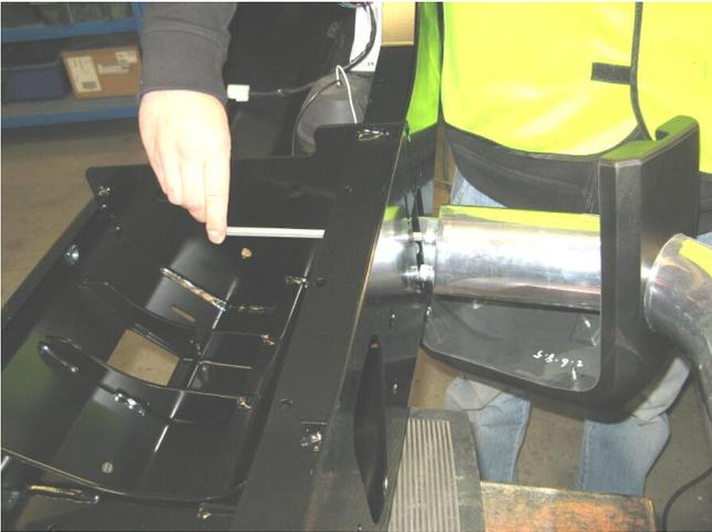
56. Fix the frame to the hinge brackets using 4 x sets M10 x 30 Cap Screws, flat and spring washers
